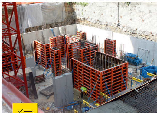
Wall Formwork - Twin Wall & Aluminum & H20 Timber Beam
